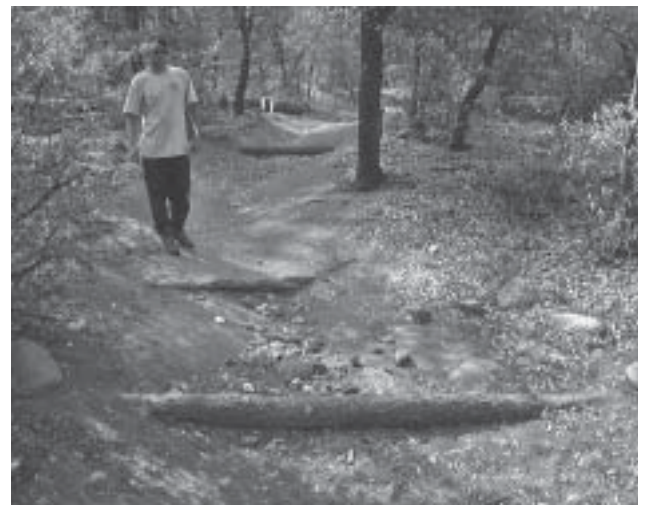
Crew member inspecting installation of water bars
